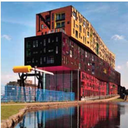
Top image - Typical kitchen Bottom image - Chips exterior
